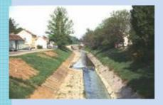
Instead of high bed-drops small structured bed – sills were installed
