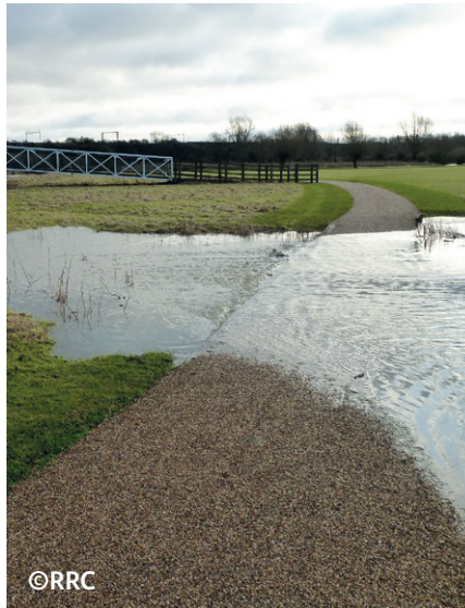
4.1km of paths, boardwalks and bridges provide full public access, some of which will be underwater during flood.
